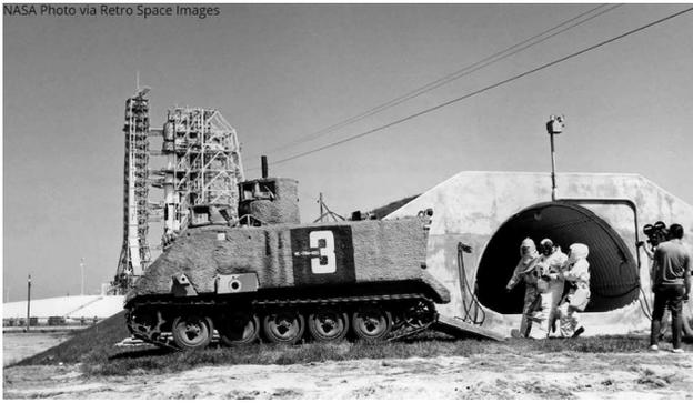
Rumbling, cramped, heavy and lacking a big field of view, the M113 wouldn't seem to be a good candidate for an ambulance. It doesn't even have a steering wheel. But it has something essential for a NASA rescue mission at the launch pad: armor.
