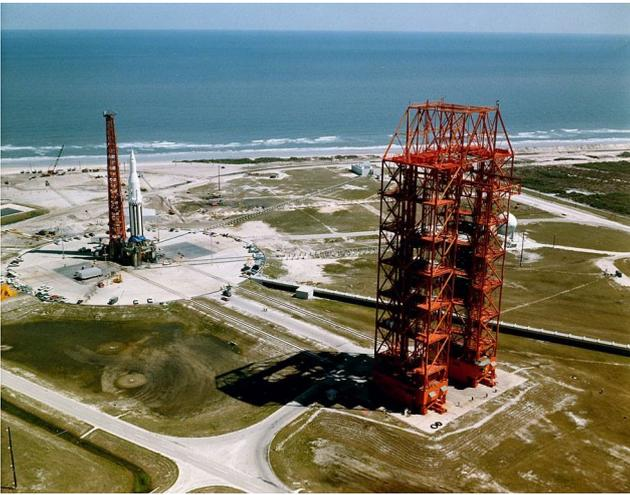
Umbilical Tower and Service Structure of LC-34 with Saturn 1 SA-4 on the launch pad.
