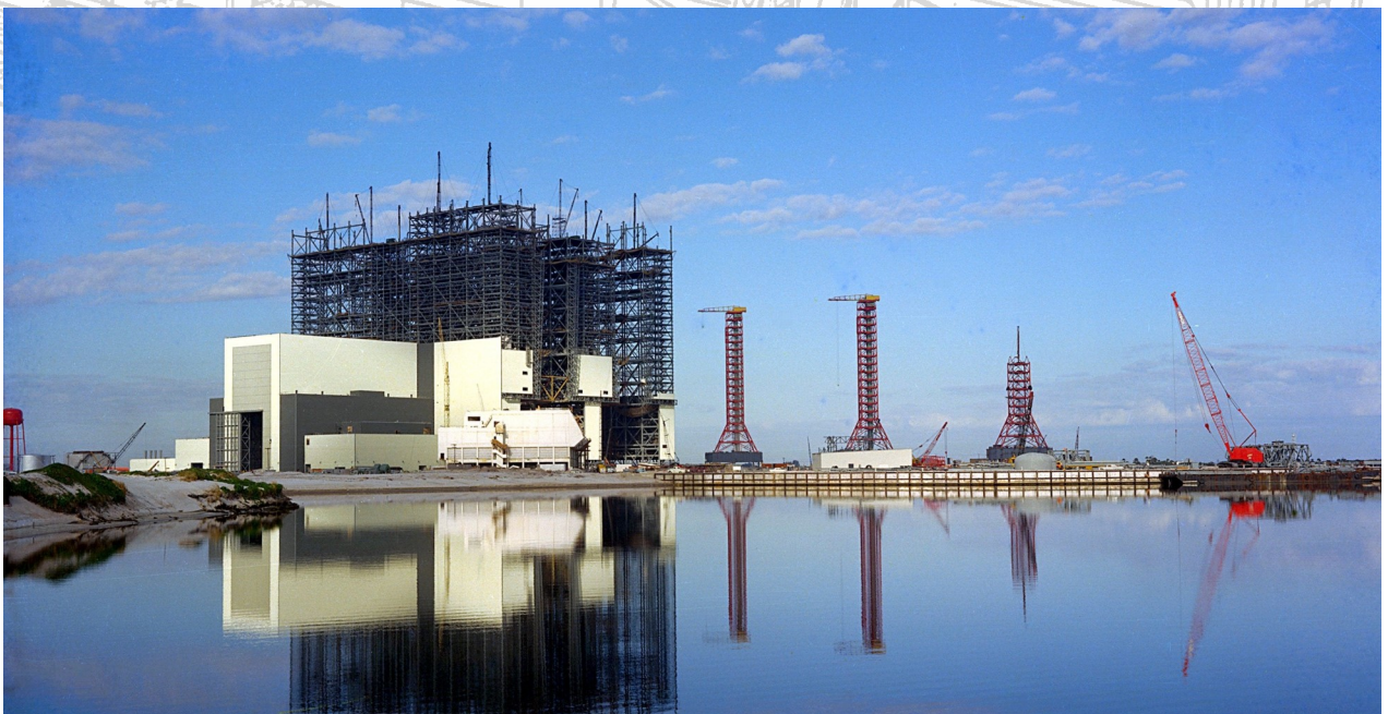
The VAB and three LUTs under construction, January 5th, 1965
