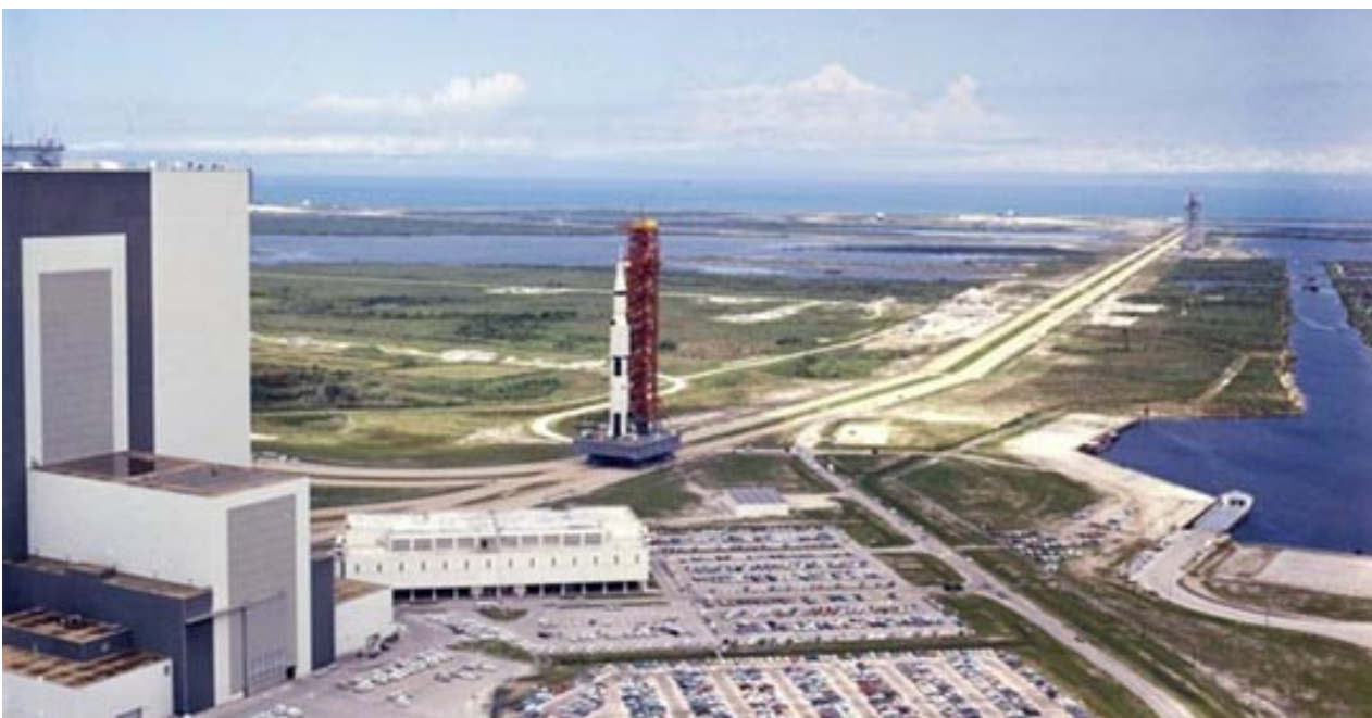
VAB, Crawlerway & Pads during Apollo 11 Rollout - 20th May 1969
