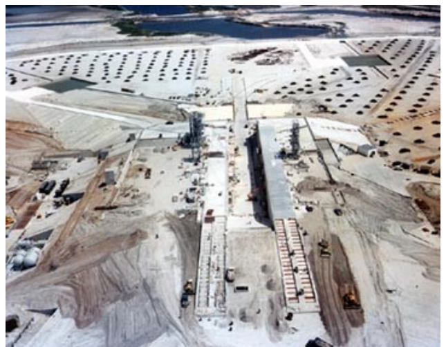
LC-39A under construction - 1st January 1965
