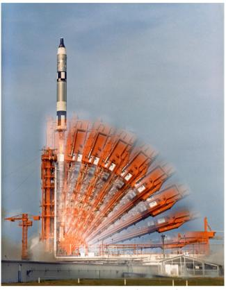
A time-lapse photograph shows the configuration of Pad 19 up until the launch of Gemini 10 on 18 July 1966. Credit: NASA
