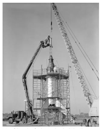
View of the mating of Little Joe-5B launch vehicle with Mercury capsule #14 on 23 April 1961. Credit NASA
